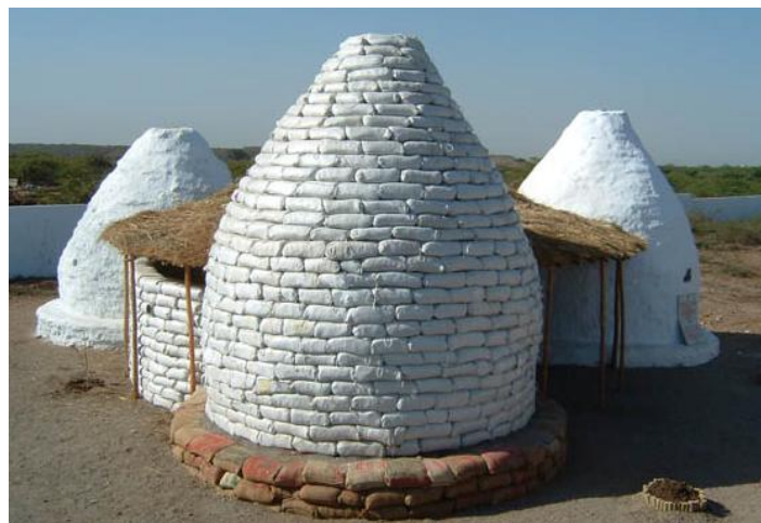
Figure 1.1: Earthbag construction project in India (Anon, 2007).
