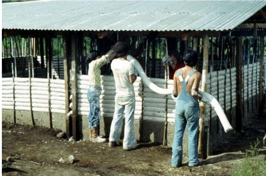
Figure 2.2: Construction of structural earthbag wall system in Guatemala, 1977 (Grasser and Minke, 1990).
