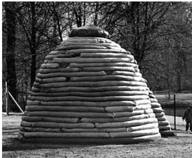
Figure 2.1: Minke's earthbag dome, built in 1977, still standing in 1997 (Grasse and Minke, 1990).
