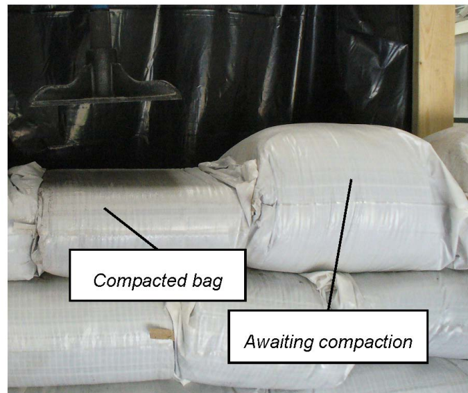
Figure 2. Earthbag compaction during wall construction.
