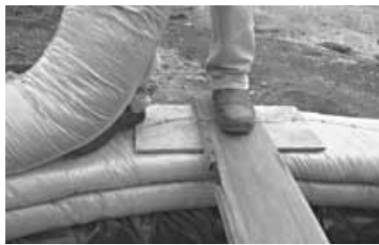
Above: Cantilevered stair treads were inserted between rows to a depth of 300mm. Right: Forms were built using scrap wood.
