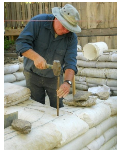
Right: Hammering rebar into bag walls.
