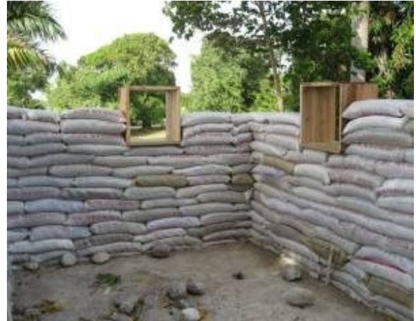
Above: Wooden window jambs in earthbag walls.
