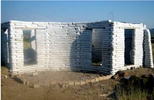
Left: Next Aid earthbag performance building.
