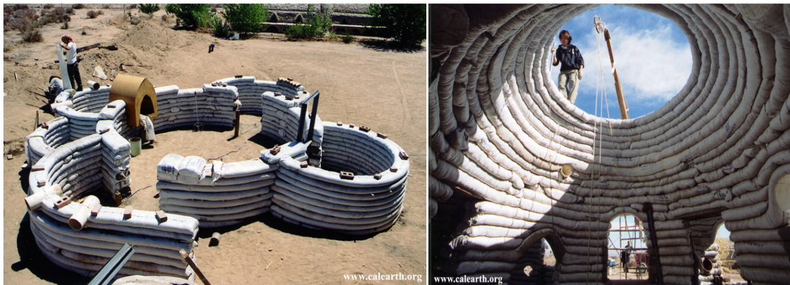
Figure 1: Construction of earthbag domes by Cal-Earth ( Cal-Earth Inc. / Geltaftan, 2010).
