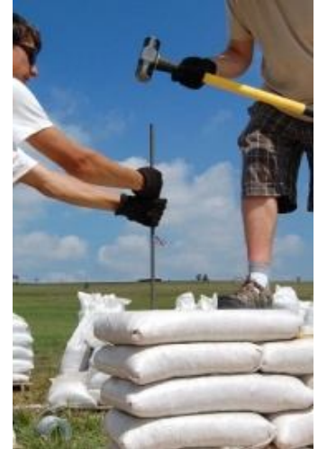
Right: Hammering vertical rebar into earthbags
