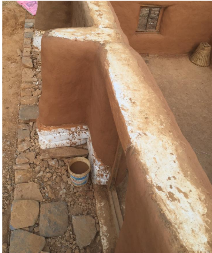
Figure 4: Preliminary plaster layers on an earthbag structure. Source : Kathryn Kaspar (2015)
