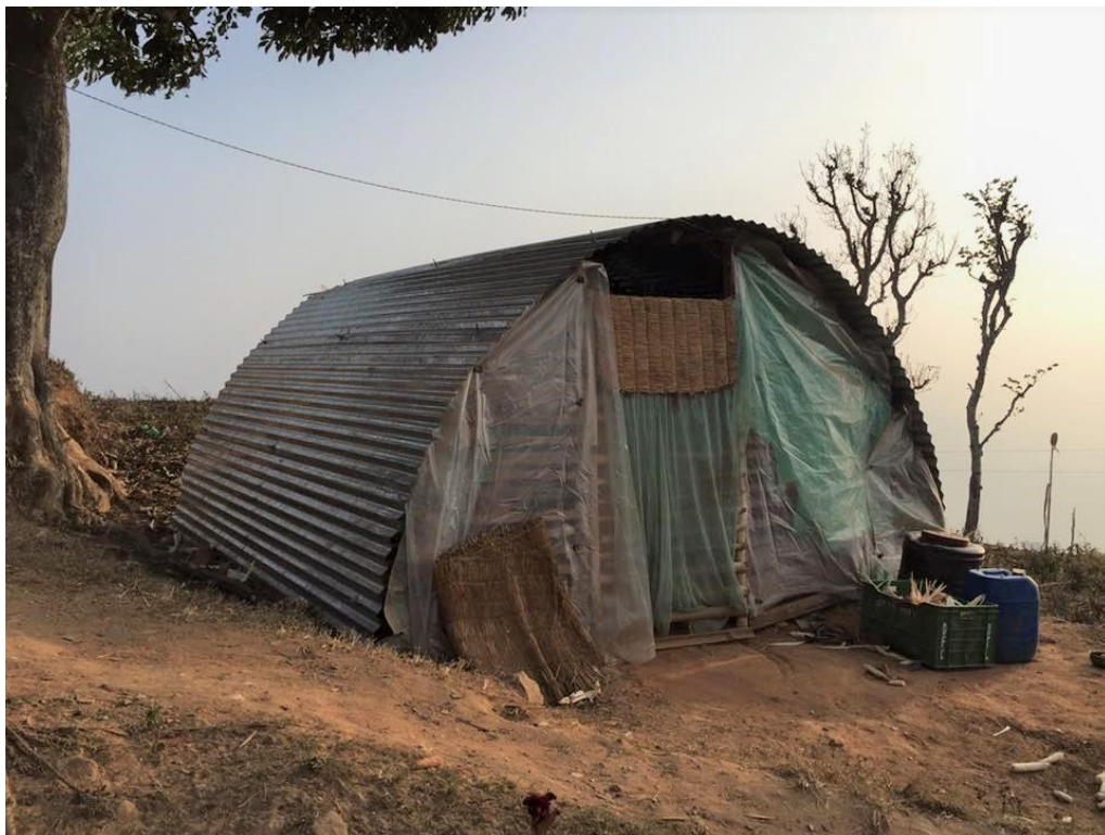
Figure 2. A typical temporary shelter in Dhading, Nepal. Source : Kathryn Kaspar (2015)
